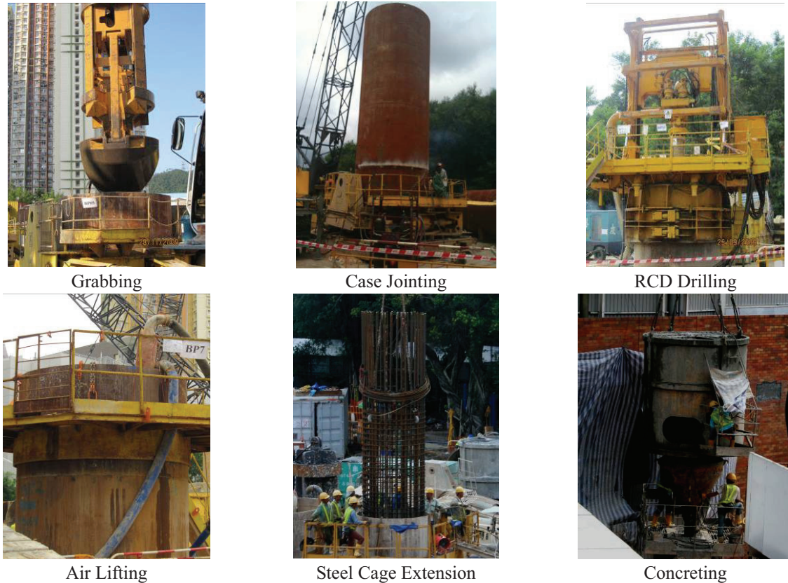
Fig. 1: Bored pile construction sequence
