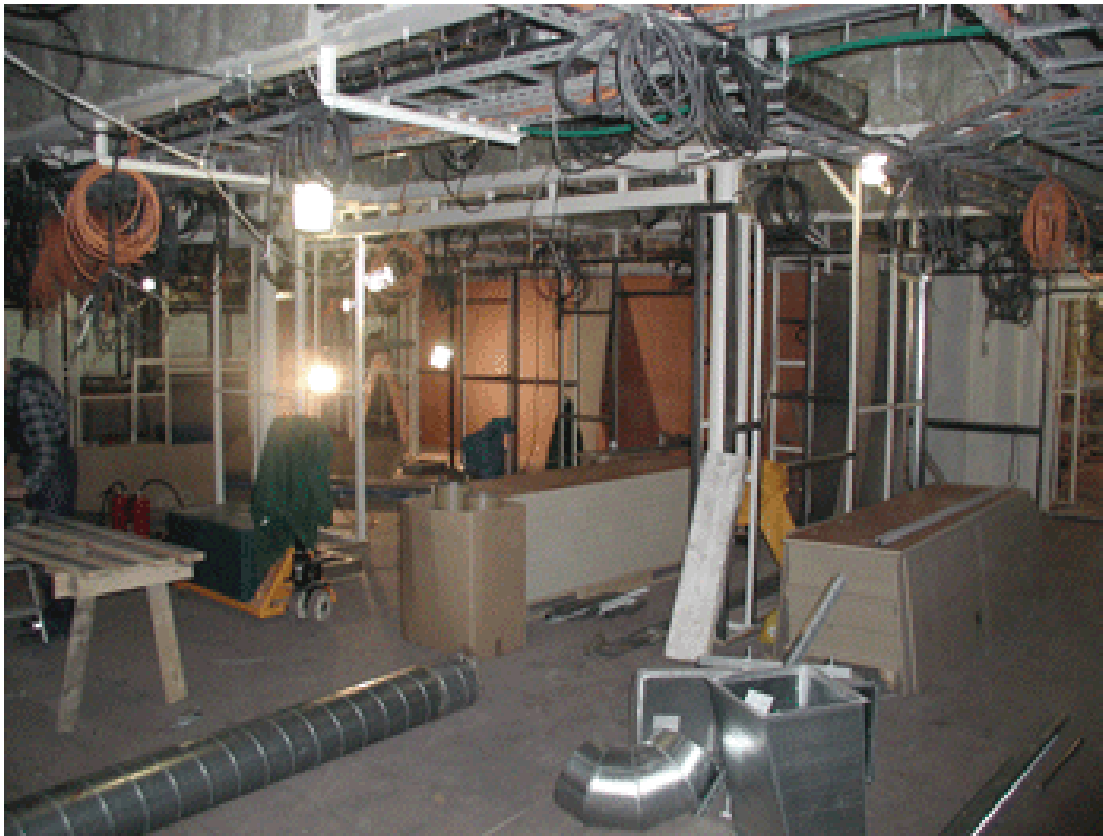
Fig. 6: outfitting processes in shipbuilding within a fire protection zone
